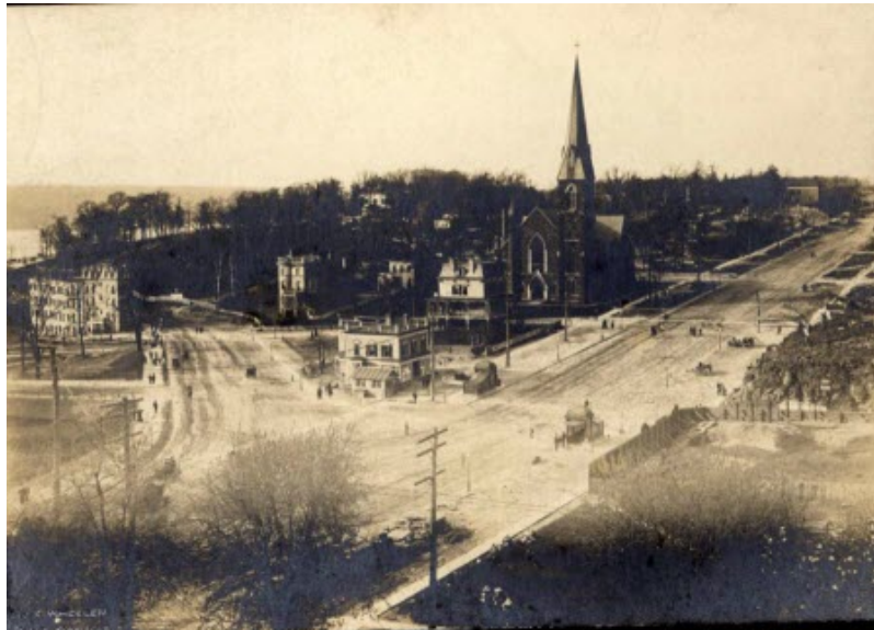
Intersection of Broadway, 156th Street, and Boulevard Lafayette where Washington Heights citizens celebrated groundbreaking for the New York subway on May 14, 1900. (Image is from 1905, when the subway was running; note the uptown and downtown entrances on Broadway.)
